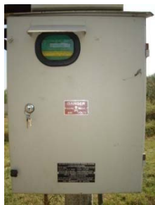
APFC system Outdoor Pole Mounted 36kVAr Contactorised Thyristorised
